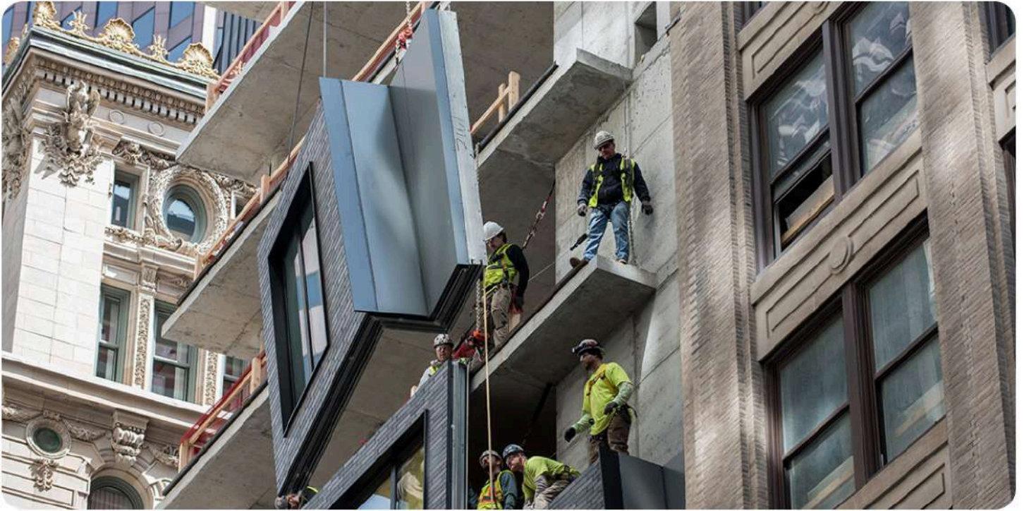
Installation of Facade system, by Redshift
