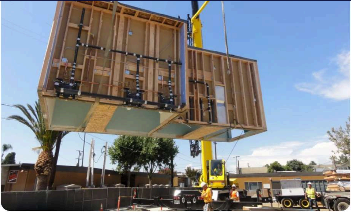
Installation of a prefabricated module, by ProjectFrog
